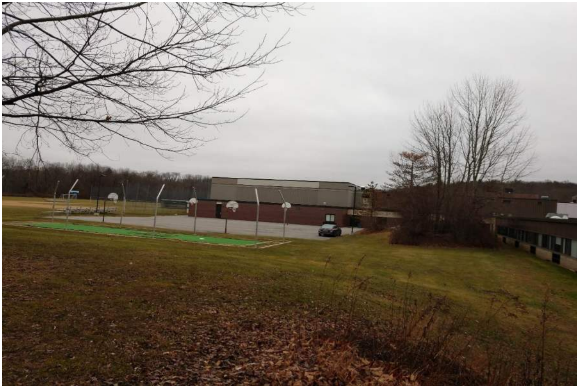
Photo 6: View to the northeast of the location of the proposed bathroom addition.
