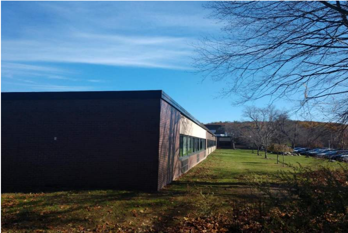
Photo 8: Pedestrian access to the new fields is currently proposed on the southwestern side of the school. View to the east.
