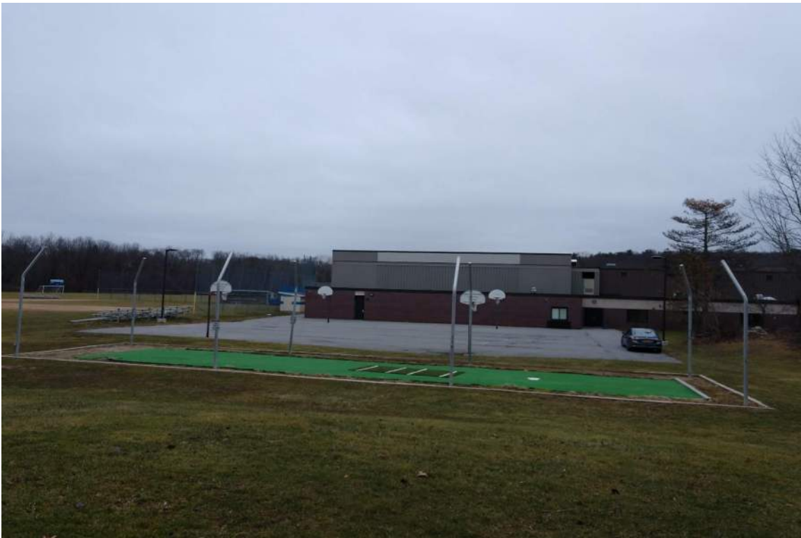
Photo 5: View to the east toward the location of the proposed bathroom addition. This portion of the school was added c. 1995.
