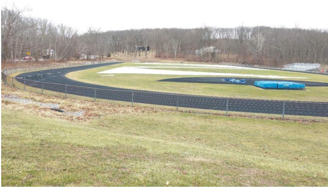
Photo 1: View to the south of Tompkins Field. Drainage culverts are located along the edge of the track.
